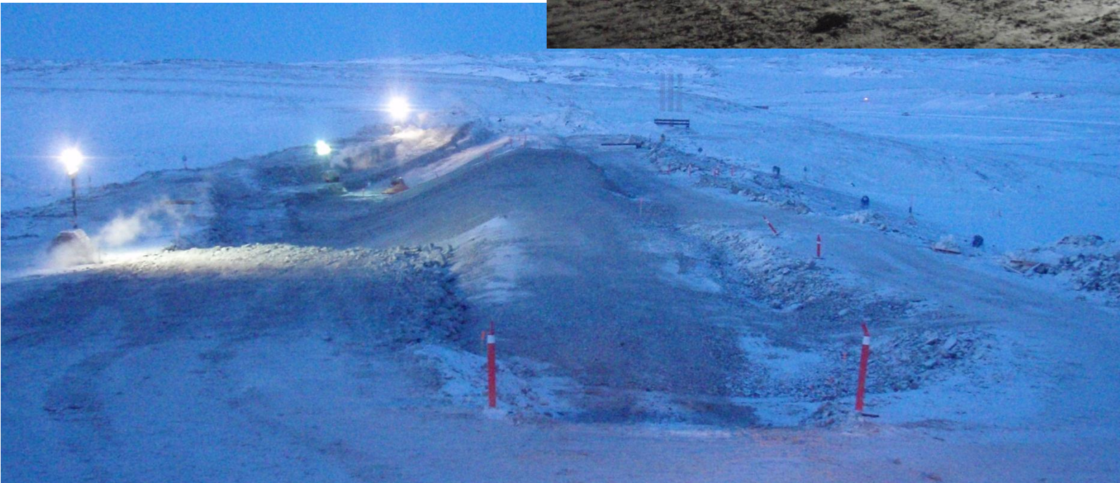
Photo 17: ~ SW view down the center of the dam. Note that the ROQ is on the left, Transition material is over the central area, the packer is working by the area where Overliner material was placed and beyond the packer to the S is the end of the GCL (around station 0+70).
