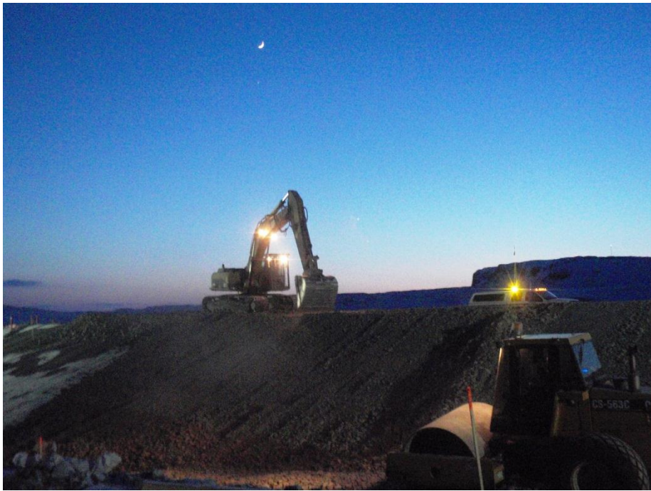
Photo 11: ~NNW view of excavator spreading Transition material placed by dayshift in a ~ 0.4m thick lift.
