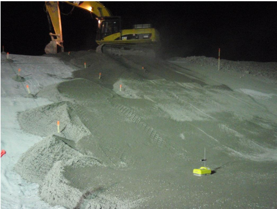
Photo 12: ~NNE view of excavator spreading Overliner (GCL cover) material. Note the density test in progress in the foreground.
