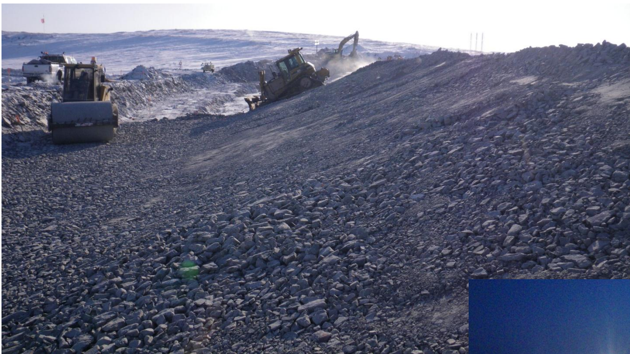
Photo 9: Transition material being placed on the slope above the liner. Photo looking south west.
