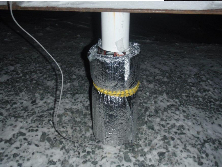
Photo 14 (bottom): Insulation wrapped around a single bead secured to the base of an exposed thermosyphon.
