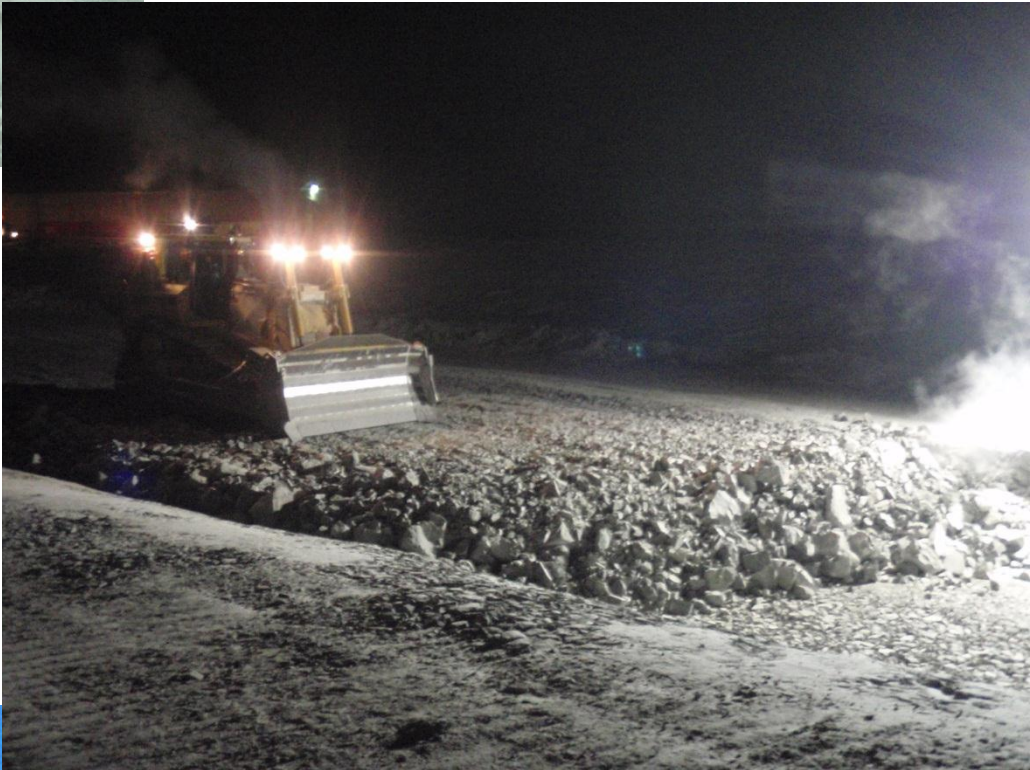
Photo 16 (right): D8 spreading ROQ at the North end of the dam (around 1+90).
