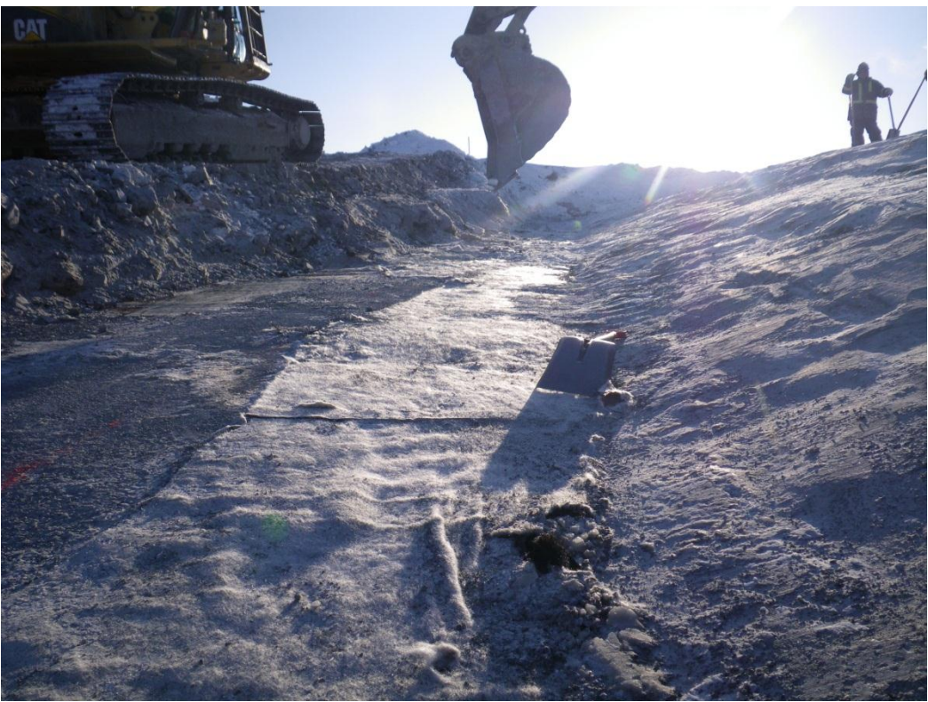
Photo 5: Holes in lower GCL near station 0+50. The hole in the foreground is right where the FCM slope meets the GCL.
