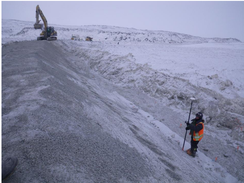
Photo 7: Survey picking up crush at base of diversion berm trench.
