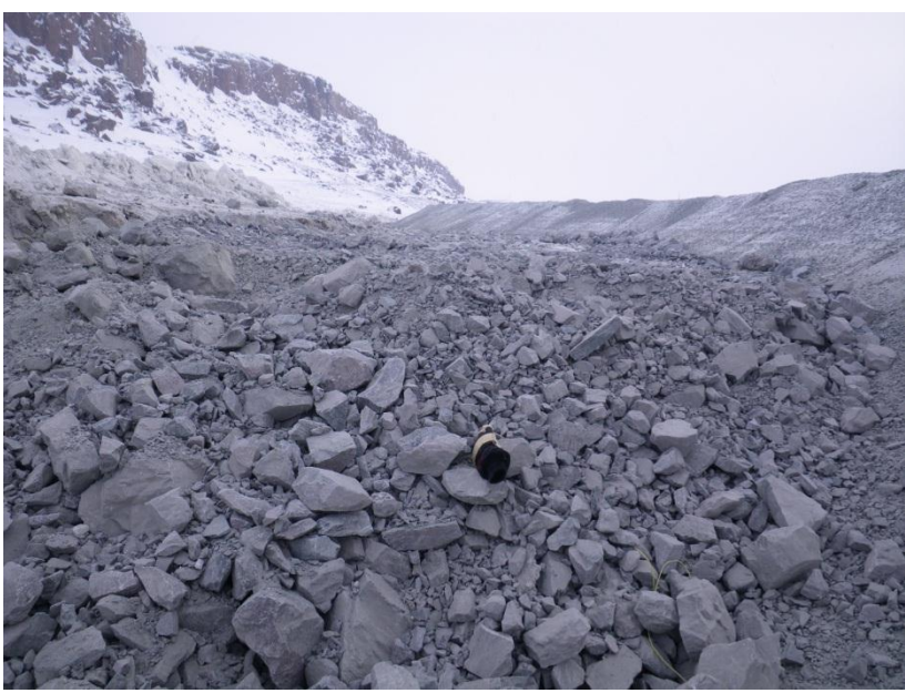
Photo 8: First lift of ROQ placed in diversion berm. The ROQ is of good quality and very fine.
